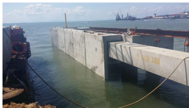
Figure 10 – Wave screen panel installation in progress
