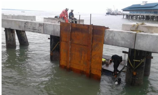
Figure 9 Dummy panel installation
